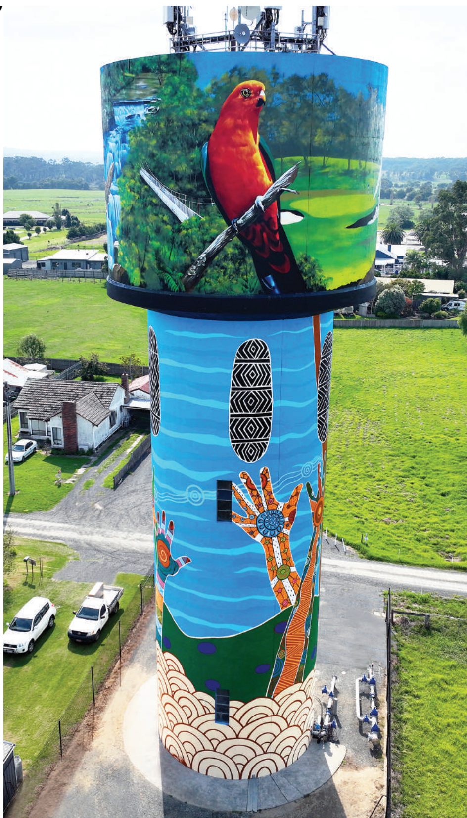
The Yarram Water Tower
