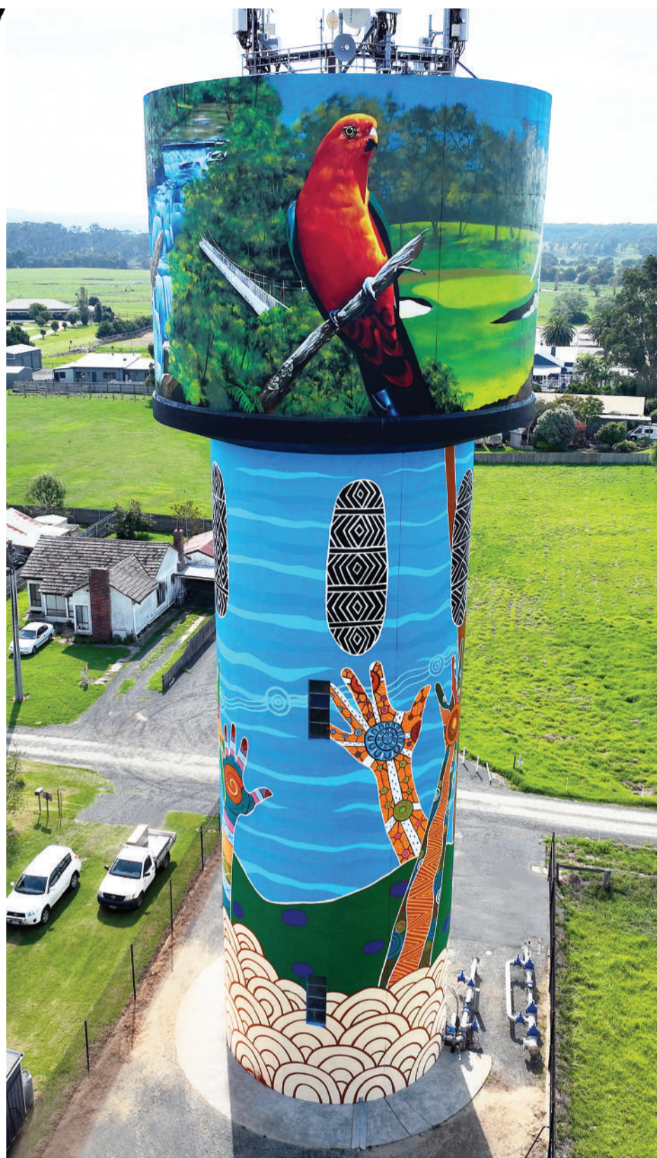
The Yarram Water Tower
